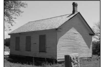
An authentic cedar shingle roof was added this summer.
